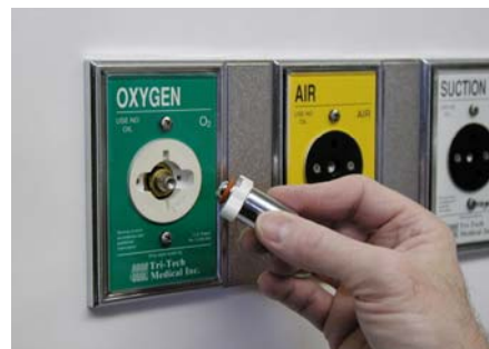
Frontall™ feature allows service of primary check valve from the front without removing the faceplate !
