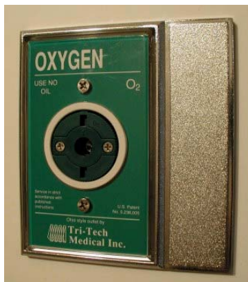
Frontall™ feature allows service of primary check valve from the front without removing the faceplate !
