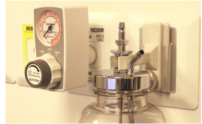
64-0603-6B with 64-0606 mounted on slide bracket with suction regulator
